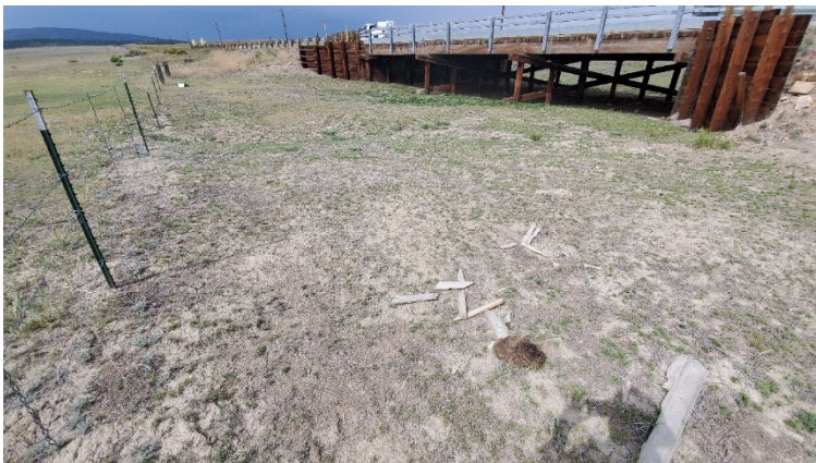
Photo 3. Wetland 1, looking southwest towards I-13-H and US 24 at part of Wetland 1 as it narrows under the bridge. Foreground is in the wetland, but area by other side of bridge failed to display wetland conditions.
